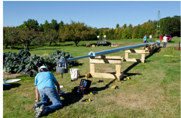
Figure 6. Example of support structure for resting the SWT when lowered (Source: Small Wind Guidebook - WINDEXchange).
